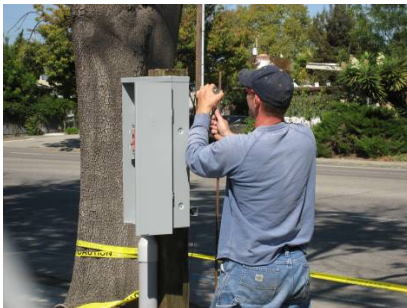
September 18 th ... Electricity on the way...
